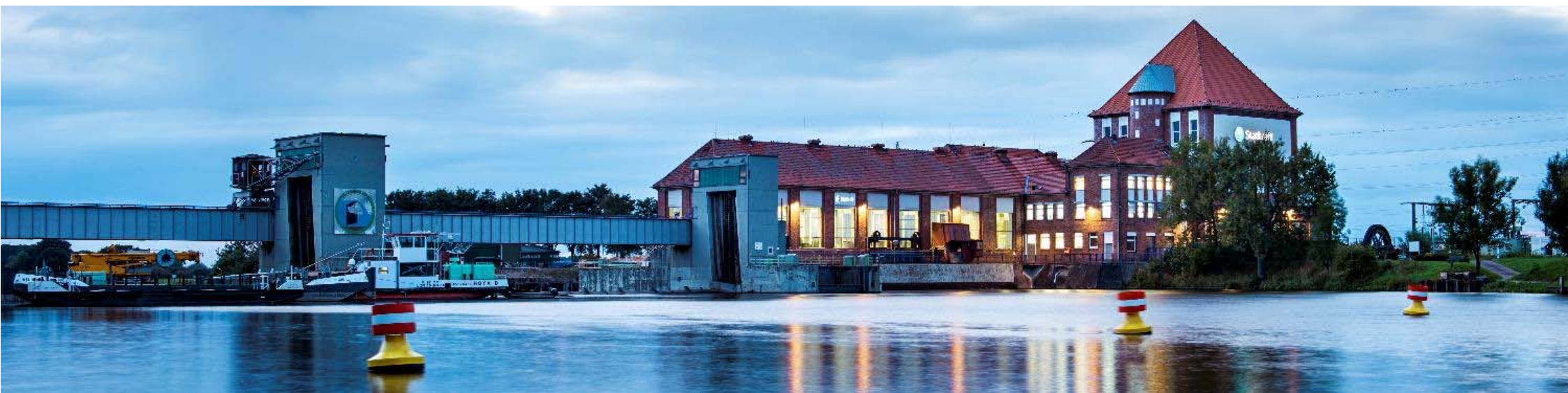
Dörverden hydropower plant, Germany
