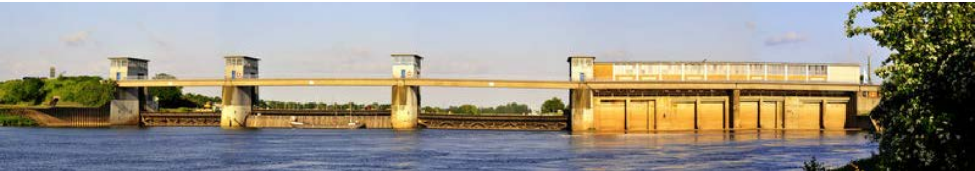
Dörverden hydropower plant, Germany
