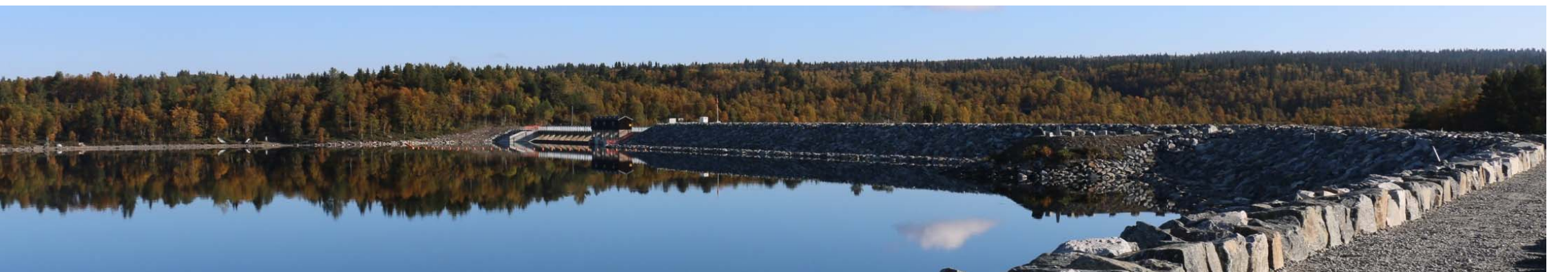
Tisleifjord hydropower plant
