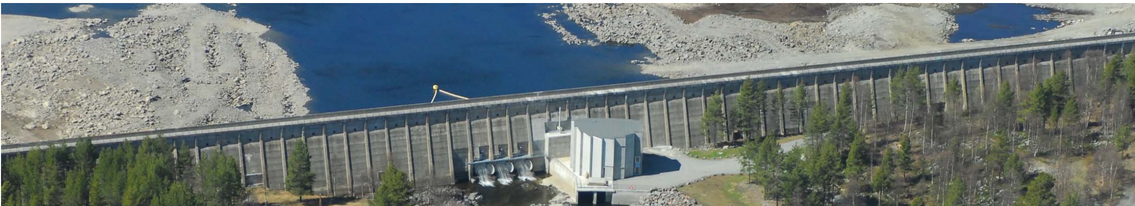
Pålssbu hydropower plant
